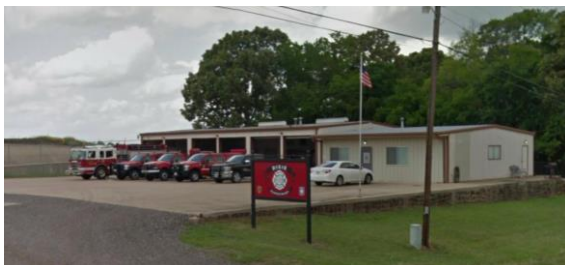
Figure 123: Dixie VFD, Station 1
